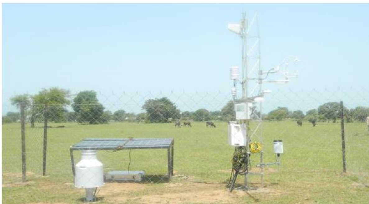
Figure 2: Installation set up at the EC station.
