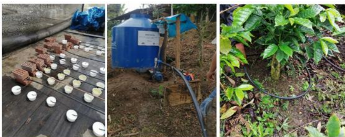
Figure 2: Left: Pilot test module for the drip irrigation system. Center: 1 m 3 tank for storage of irrigation water. Right: Irrigation system installed in final field
